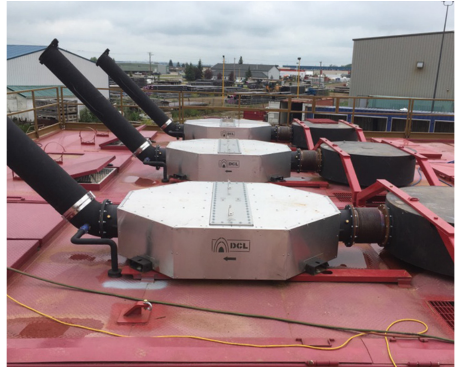
Muffler boxes installed on the rig generators to dampen the noise.
