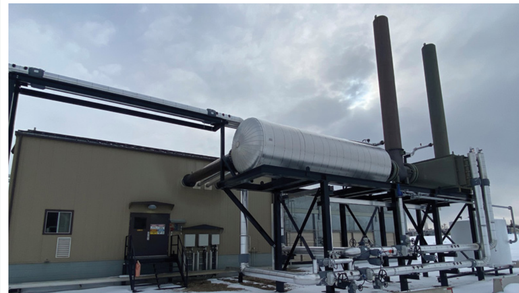
New waste heat recovery unit installed on the PK5000 compressor at Phase I/II of the Pouce Coupe Gas Plant
